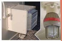
Explosion-proof interior light with UL listed exterior on/off switch. Explosion-proof mechanical ventilator tied to light switch for forced vapor removal at 750 CFM. Explosion-proof conduit and wiring with seal-offs.
